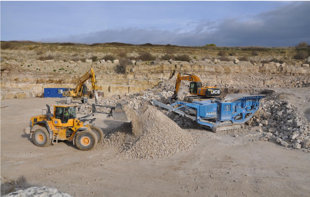
Plate 1: Crushing and Screening operation
